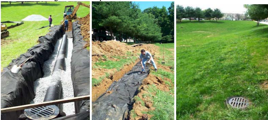
Figure 4: Example of Infiltration Trench Installation
